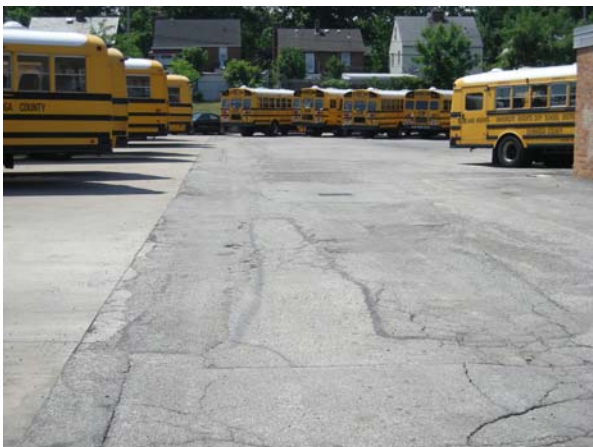
Deteriorated Asphalt
