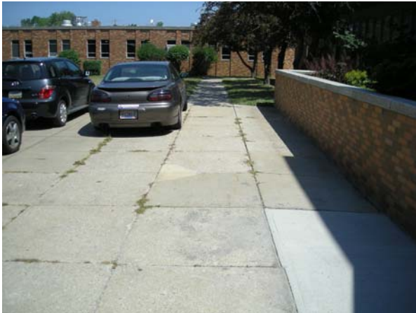
Parking at Concrete Paving
