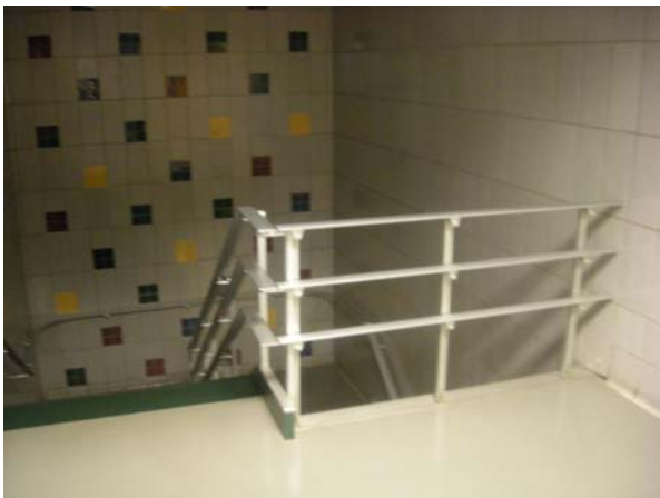
Typical Handrail at Stair
