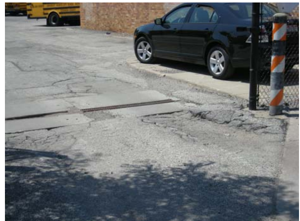
Deteriorated Asphalt
