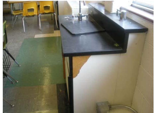
Peeling Laminate at Science Casework
