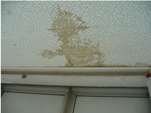
Water Damaged 12x12 Ceiling Tile
