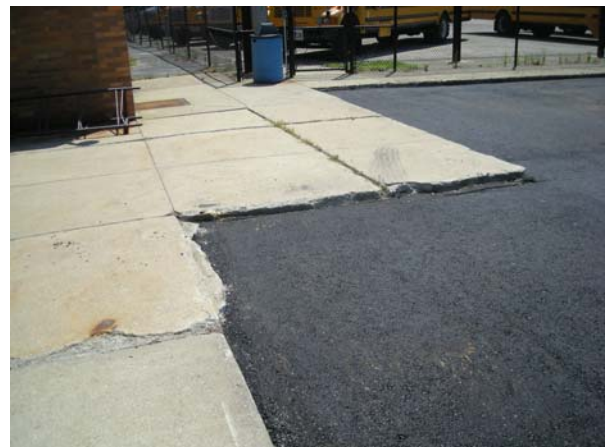
Deteriorated Concrete Walk
