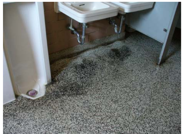
Stained Terrazzo at Toilet Room
