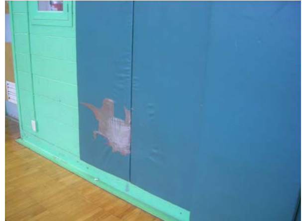
Damaged Gymnasium Wall Pads
