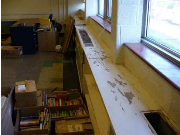
Peeling Paint at Casework Below Window
