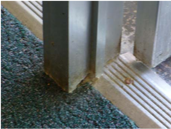
Corrosion at Bottom of Aluminum Frame
