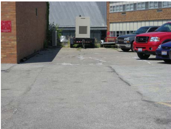
Deteriorated Asphalt
