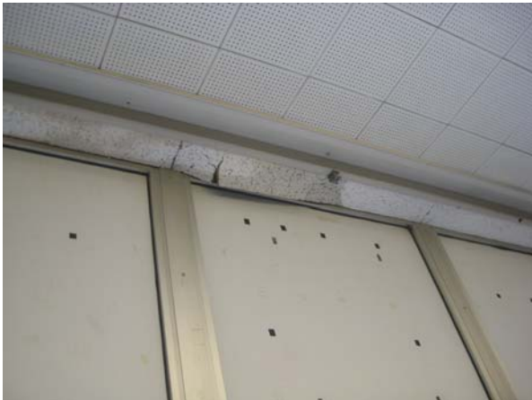
Deteriorated Tile at Window Head
