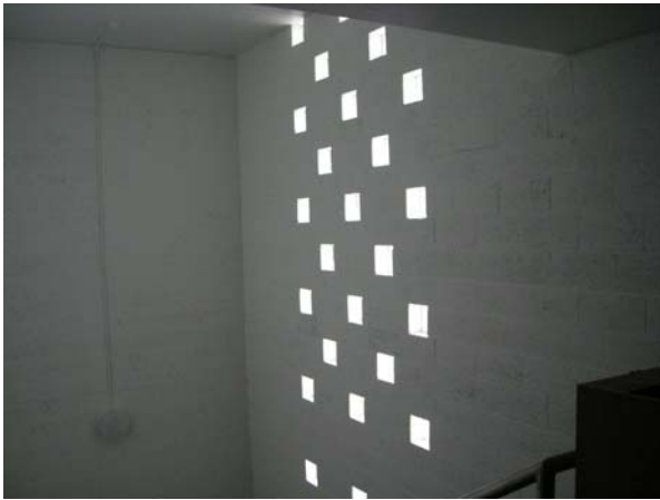
Glass Block at Stair
