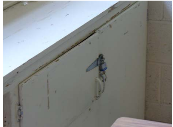
Casework Below Window
