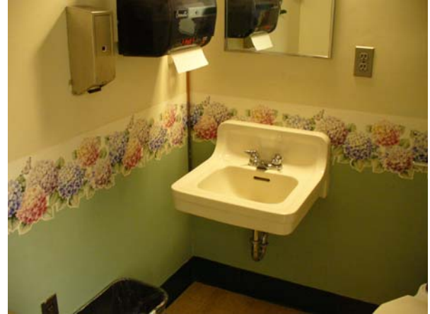
Staff Toilet Room
