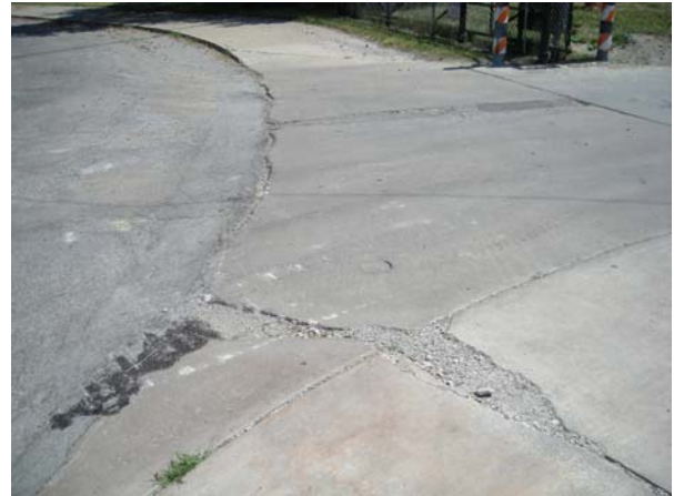
Deteriorated Concrete Drive
