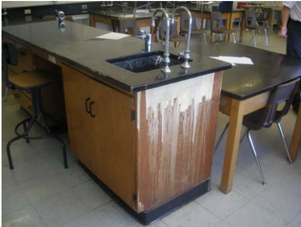
Damaged Science Casework and Table
