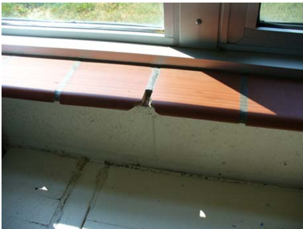
Crack at Tile Sill
